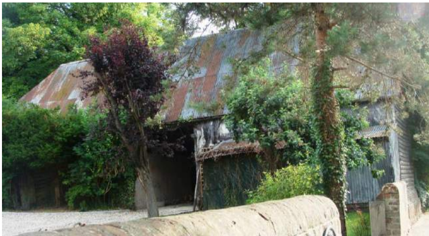
Picture 45. Grade II barn at Little Meadow, the corrugated roof was originally thatch. A thatch replacement roof would represent a significant gain. Potential grant assistance may be available. The building is on the Council's Heritage at Risk Register.
